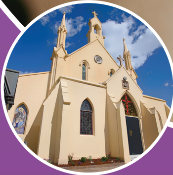
Saint Francis Xavier Cathedral 36 Harbour Street Wollongong
